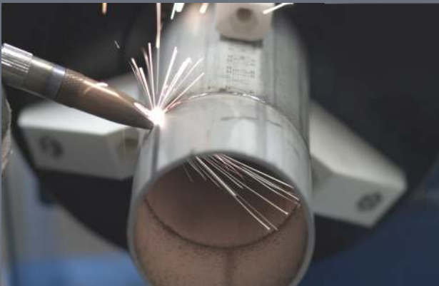
CREATING COMPLICATED JOINTS
