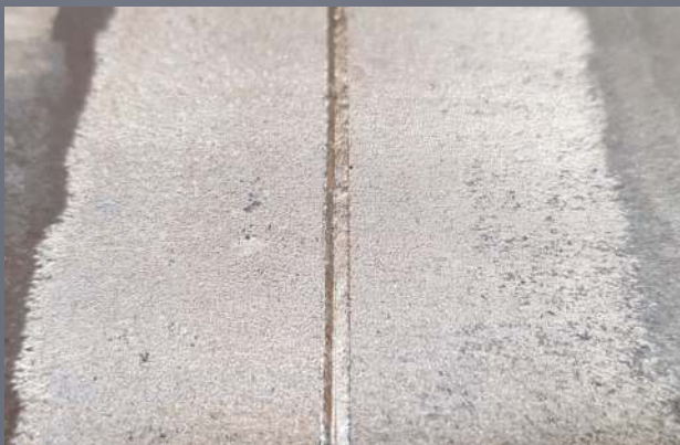
WELDING OF LARGE AND THIN STEEL PLATES
